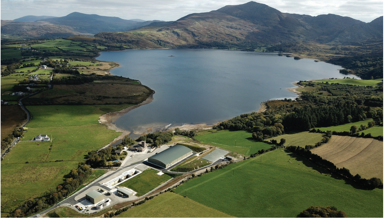
New Kerry Central Regional Water Treatment Plant at Lough Guitane opened in November, 2019
