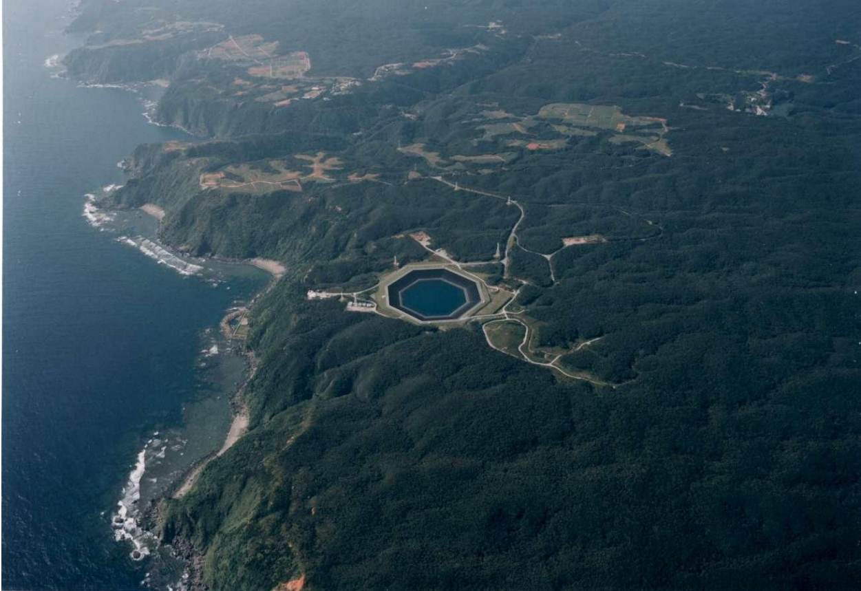
Figure 2: 85MW Seawater Scheme with an Artificial Upper Reservoir has been Operating at Okinawa, Japan
